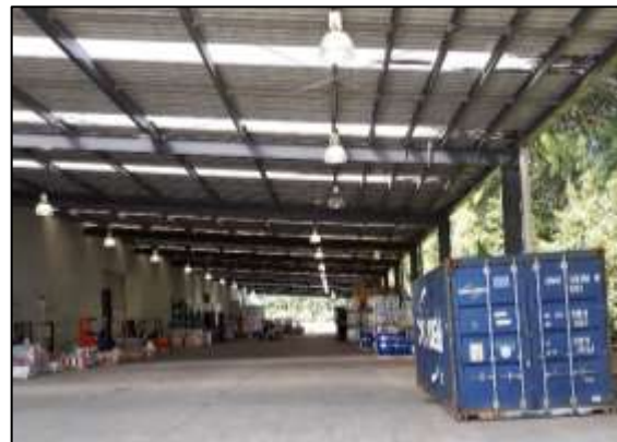
Figure 4: Transit Depot Canopied area
