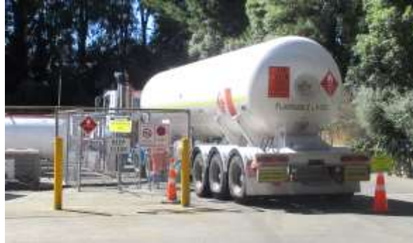
Figure 5: LPG tanker delivery underway just outside the canopy area
